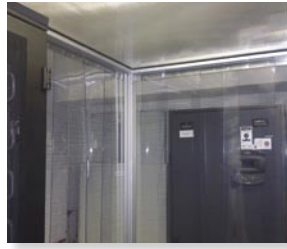
Hot and cold air is separated using containment.
