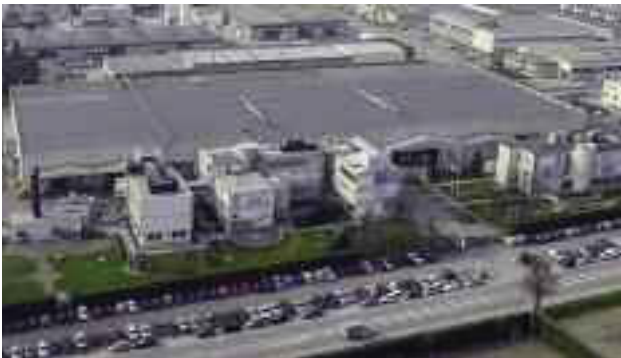
Emerson Network Power Headquarters EMEA
